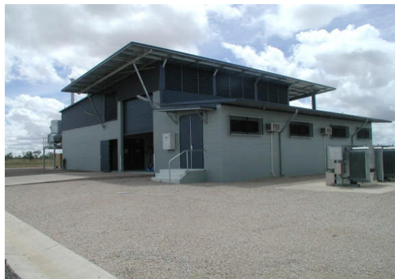
Rural Community Power Station [Ergon Energy, Australia]
