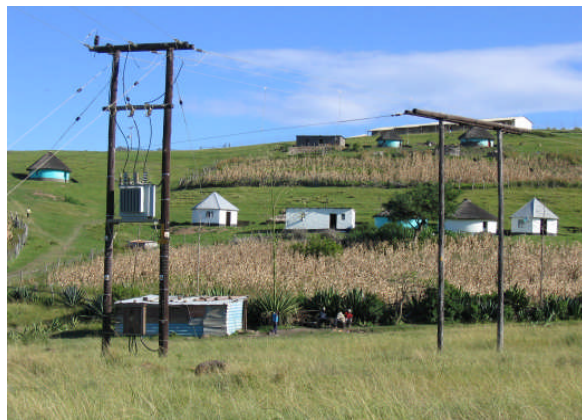
Rural electrification in South Africa [C.Young]
